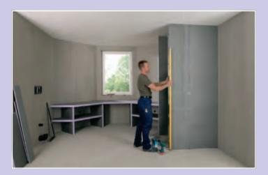
The shower partition wall is finished. Prior to laying the tiles, all of the board joints outside the shower must be filled with JACKOBOARD glass fibre tape.
