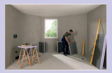
The construction board elements are glued to the wall and floor to provide the substructure for the washstand.
