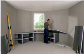
The washstand top is glued to the substructure. Prior to tiling, all of the board joints and visible top edges are filled with JACKOBOARD glass fibre tape.
