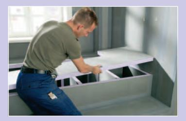
JACKOBOARD Plano is cut to the right shape and glued onto the supporting structure as a panel using assembly adhesive.
