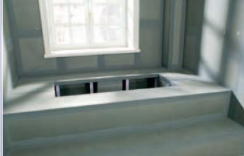
The bathtub can then be positioned in the recess. The pre-fabricated JACKOBOARD Wabo bathtub element is an alternative product that can be used for simple, vertical bathtubs.
