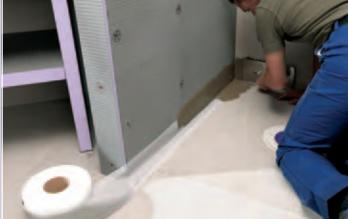
To avoid water dripping down the back, all of the joints and transitions in the wet area of the shower must be sealed with JACKOBOARD sealing tape.
