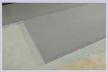
JACKOBOARD Plano is aligned and straightened with the help of a spirit level.
