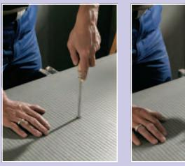
When using JACKOBOARD Plano for wall applications, a screwdriver is used to punch 8 holes (5 per m<sup>2</sup>) through the board for marking purposes. Dabs of mortar are then applied over these hole markings.
