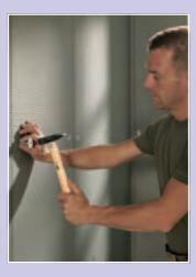
Once the mortar has hardened, a hammer drill is used to drill the dowel holes and the board is fixed with JACKOBOARD metal plugs. Again, the hole markings help when drilling the holes.
