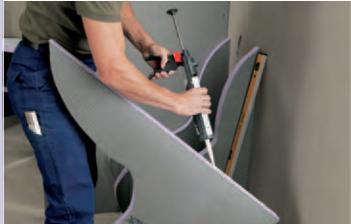
The substructure for the bench is made of 50 mm JACKOBOARD Plano that is cut to shape with the help of a jigsaw.
