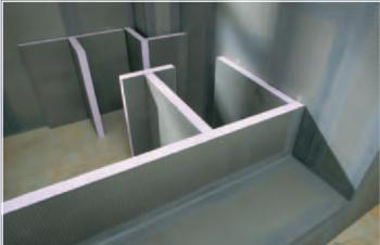
Additional board retaining walls are glued to the wall and floor at a distance of about 40 cm using assembly adhesive.
