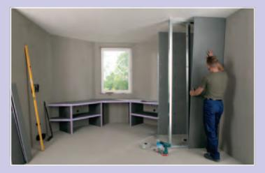
The JACKOBOARD Aqua shower element is already installed at ground level with the screed. The metal stud frame forms the substructure; the JACKOBOARD Plano construction boards are cut to the right length.
