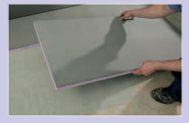
To compensate cracks and provide additional thermal insulation in floors, the construction board is moved back and forth gently to embed it firmly in the tile adhesive.
